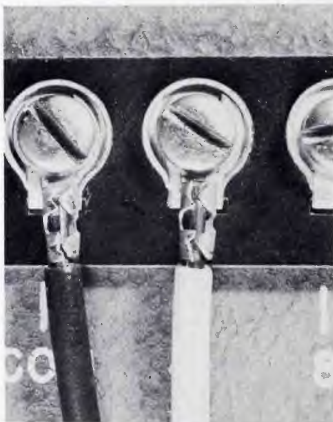
Fig. 1 The terminal connectors shown here are crimped to the wires. This is an especially hazardous practice if the wires are copper. Creeping corrosion inside the clamp is possible.
